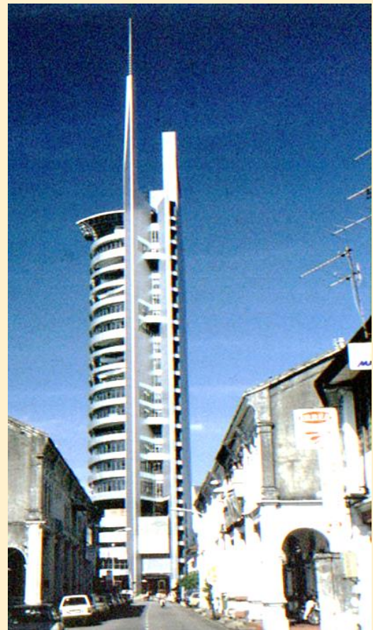
Figure 10: View showing the wing walls in the southwest and the 'air-lock balconies' (Source: Salib and Wood, 2012)
